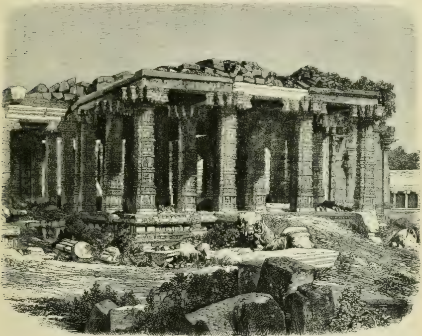
RUINED TEMPLE OF CHILLAMBARAM.
